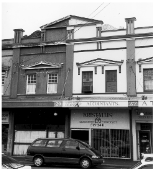
Figure 18 Inappropriate paint schemes on adjacent lots comprising part of a 'row' building detract from appreciation of the building's unity
